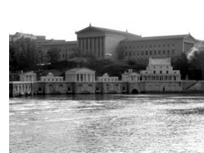
Water Works Gardens
